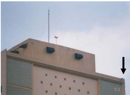
Figure 4: A photograph of the Wisma Tanah building taken in 2003. The building had been struck by lightning as can be seen on the right.
