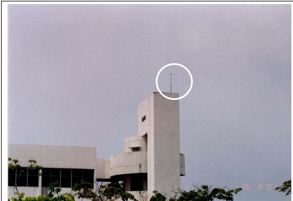
The SIRIM Block #8 with the ESE air terminal (circled) that was installed between January and August 2001. SIRIM still continued to install the ESE air terminals even though the ESE technology had just been dropped from the new Malaysian standard.
