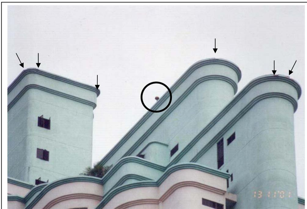
The Villa Putri apartment building in Kuala Lumpur was damaged (arrowed) by lightning at 7 different places on the roof. In spite of this building being a subject in a conference paper in 2000, the sales engineer still informed the building manager in 2002 that the building was free from lightning strike damages. One of the two Australian ESE air terminals can be seen above (circled).
